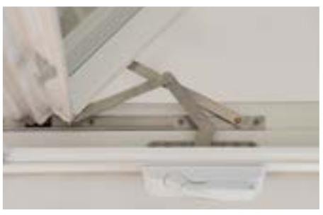
Stainless steel operator, hinge track, and hinge arm
